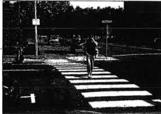
Zebra (aka Continental) crosswalks are more visible to drivers than standard double lines.
